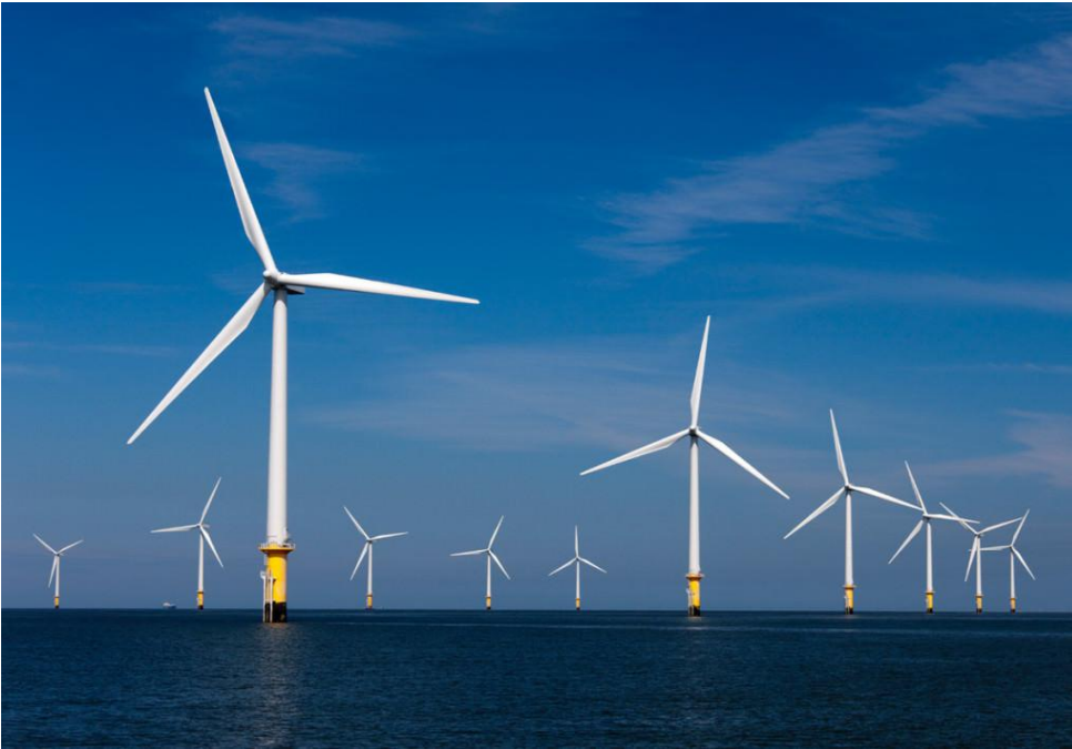
HAWT 10 MW wind farm project from Siemens (above)
